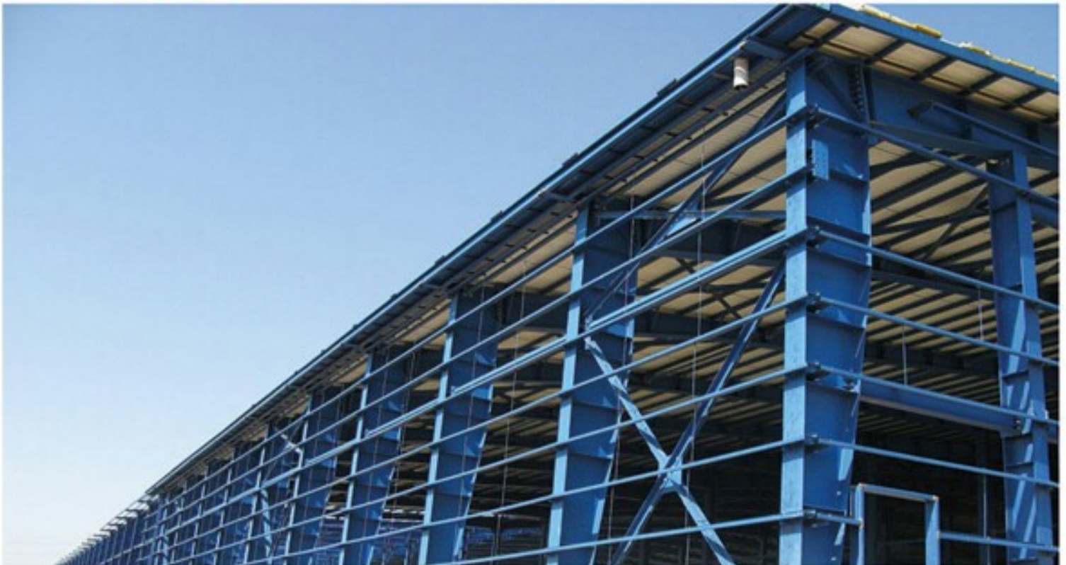
Fabrication and Erection of Molfix Hall in Pars Hayat Company / 3200 TON
